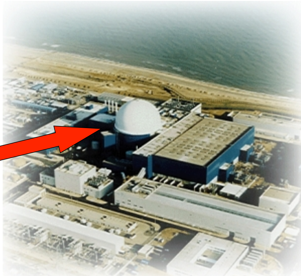
Sizewell B Nuclear Power Station
